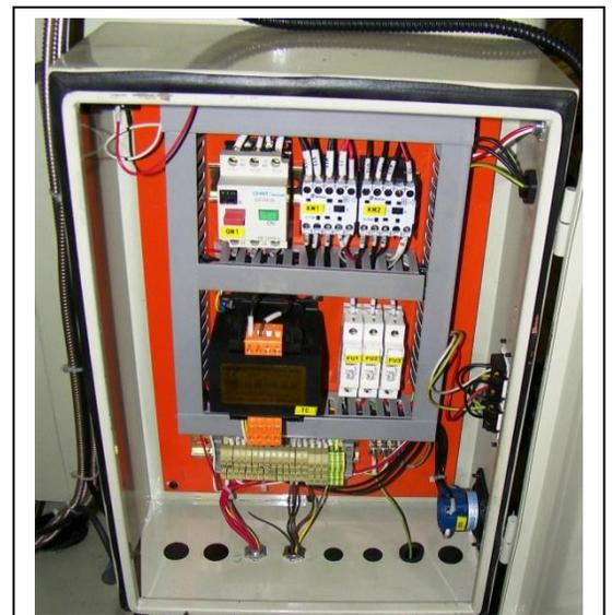
Electrical Cabinet –Control and accessory power transformer, circuit breakers and main disconnect.
